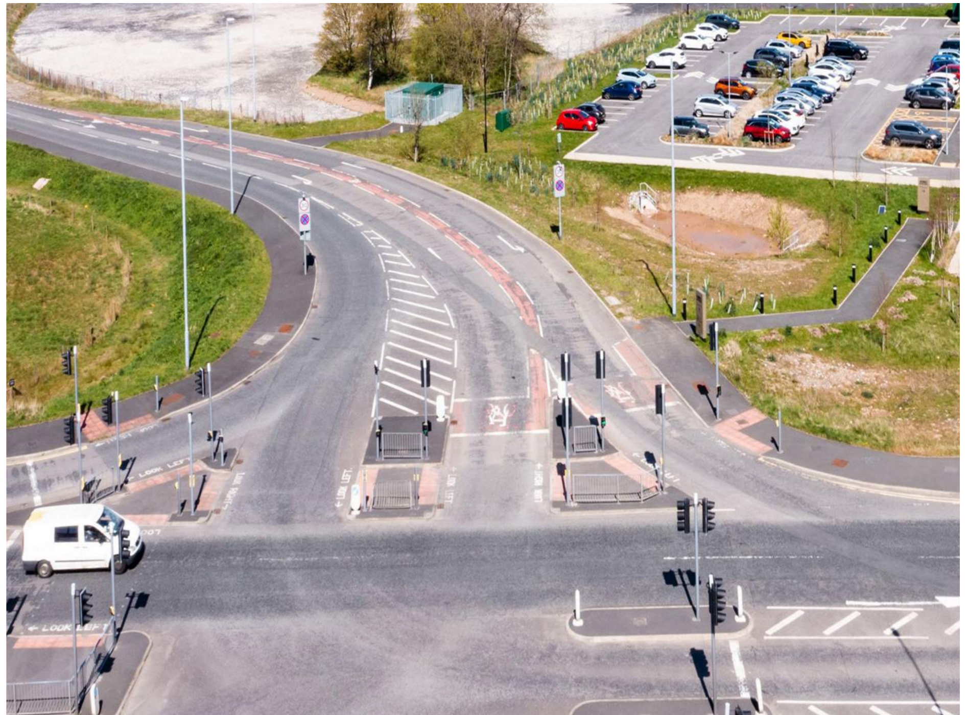
Fig. 34 - Existing photograph of the A677 junction.
