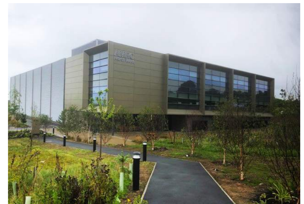
Fig. 30 - Completed landscaping within plots.
